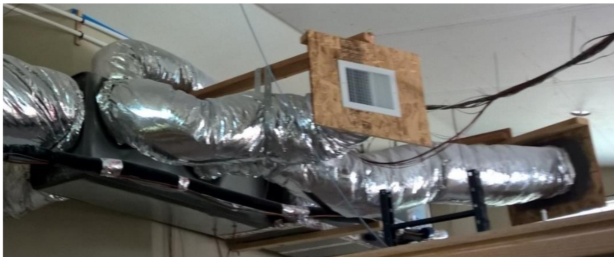
Figure 5. Duct system entirely within conditioned space.
