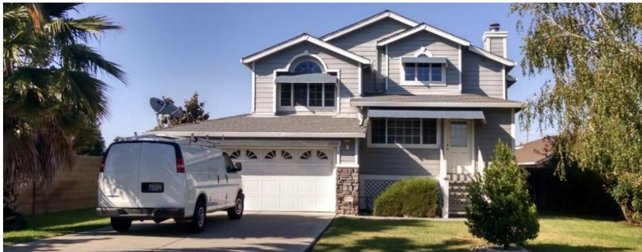
Figure 1. CVRH Radiant House.
