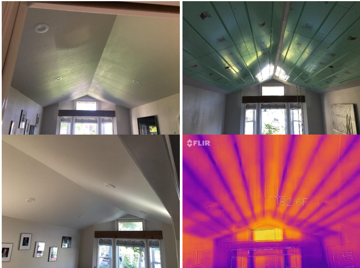
Figure 6. The great room from upper left to lower right: pre-retrofit, panel installed, finished retrofit, post-retrofit thermal image.
