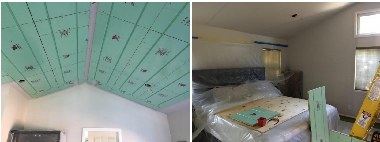
Figure 5. The installation of the radiant panels was somewhat disruptive and required the homeowners to leave the house unoccupied during the weeks of installation. The panels were mounted on the outside of the existing ceiling drywall (left). Furniture and flooring were protected during the installation (right).
