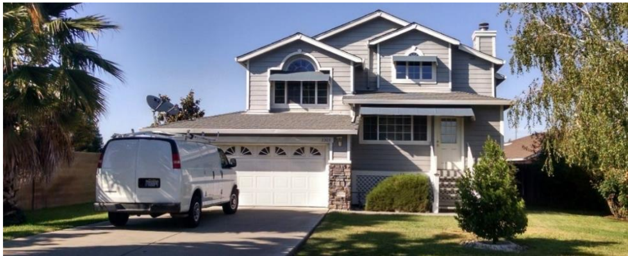
Figure 2. CVRH Radiant House.
