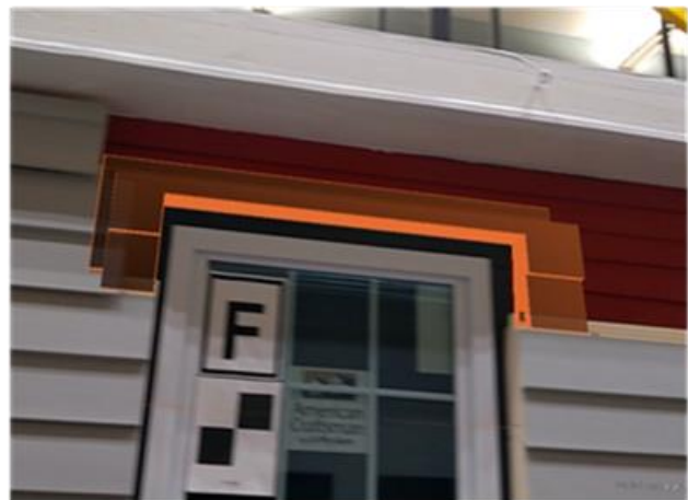
Figure 8. AR highlights for the worker the next PB to install (left) and, when prompted, shows where to install it (right; note that the PB highlighted on pallet differs from that projected on the wall).
