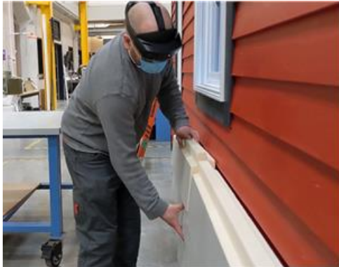
Figure 7. Worker using the Microsoft Hololens headset to install insulated panel blocks.
