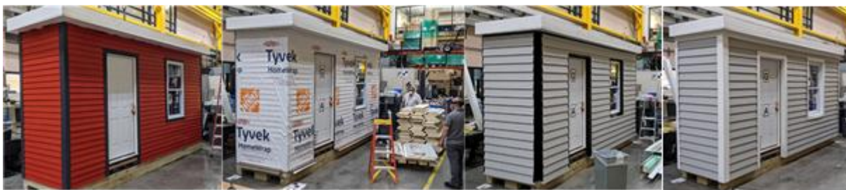
Figure 11. Sequence of steps for installing the panel-block system on the mock-up wall from left to right: 1) Pre-retrofit; 2) WRB installed and taped; 3) PBs installed and joints taped; and 4) Trim pieces installed.
