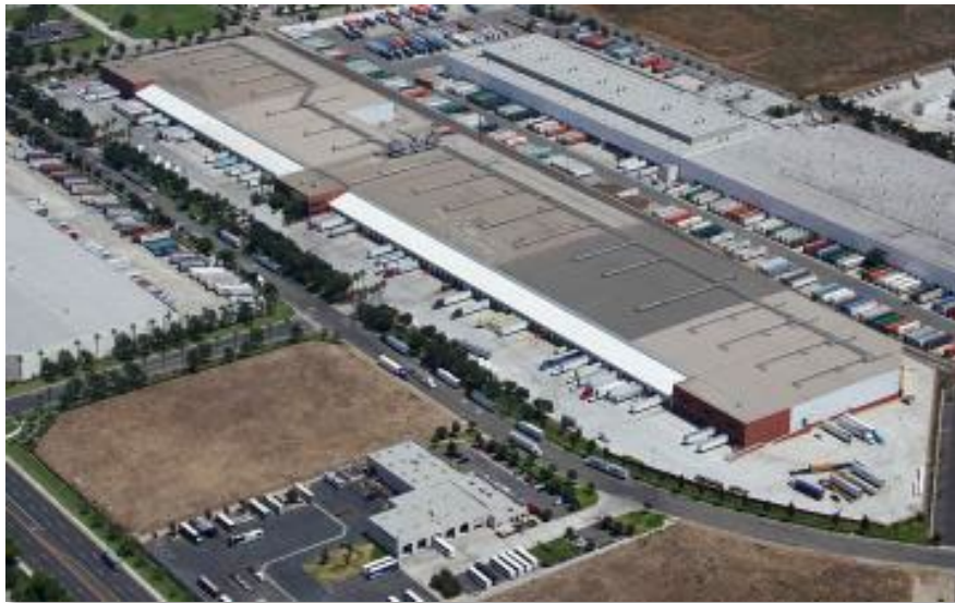
Figure 1: Aerial view of the 65,000 m 2 facility that hosted the demonstration discussed in this paper. Refrigerated semi-trailers loading and unloading at the dock are clearly visible. Source: Lineage Logistics 2021.
