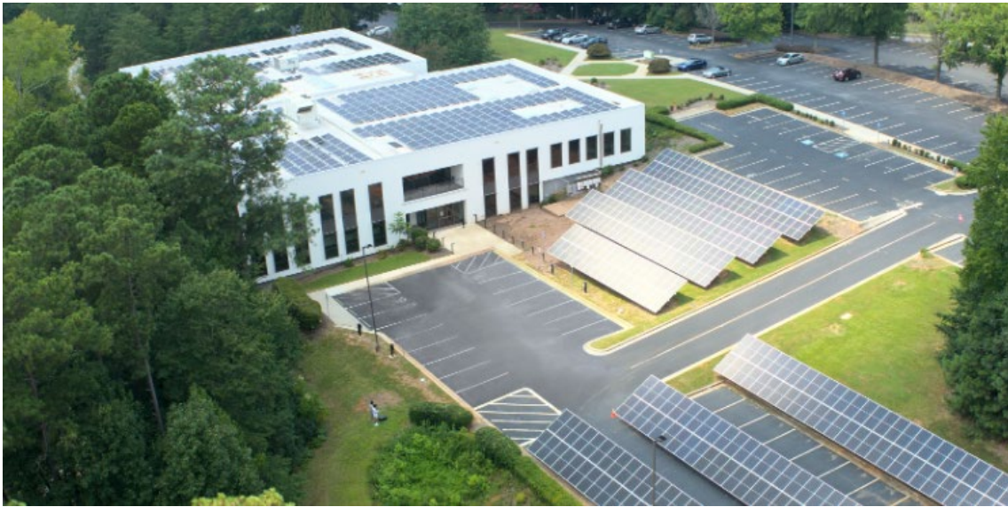
Figure 1. The renovated ASHRAE HQ building with PV system installation was completed in October 2021. Source: ASHRAE
