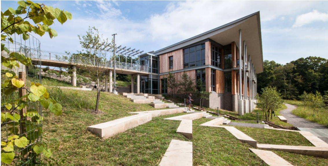
Figure 2. Frick Environmental Center image to be updated by Lawrence Berkeley National Laboratory. Source: Pittsburgh Parks Conservancy and the Greenspace Alliance, Jeremy Marshall
