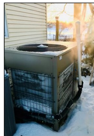
Figure 8: Comparison of AWHP "GasHP Combi" with other options in Chicago (left); GasHP Combi at -5F ambient temperature (right). Source: GTI Energy
