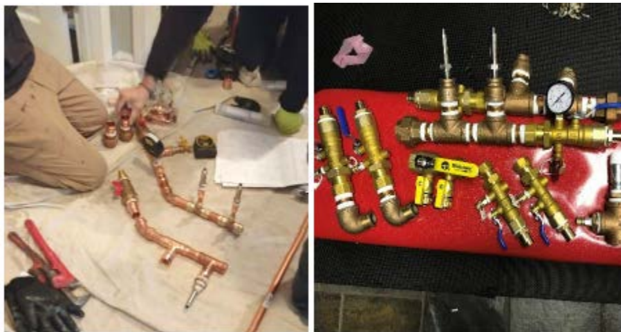
Figure 6: Manual plumbing assembly at early site (Left) and pre-fabricated/assembled fittings for later site (Right) Source: GTI Energy
