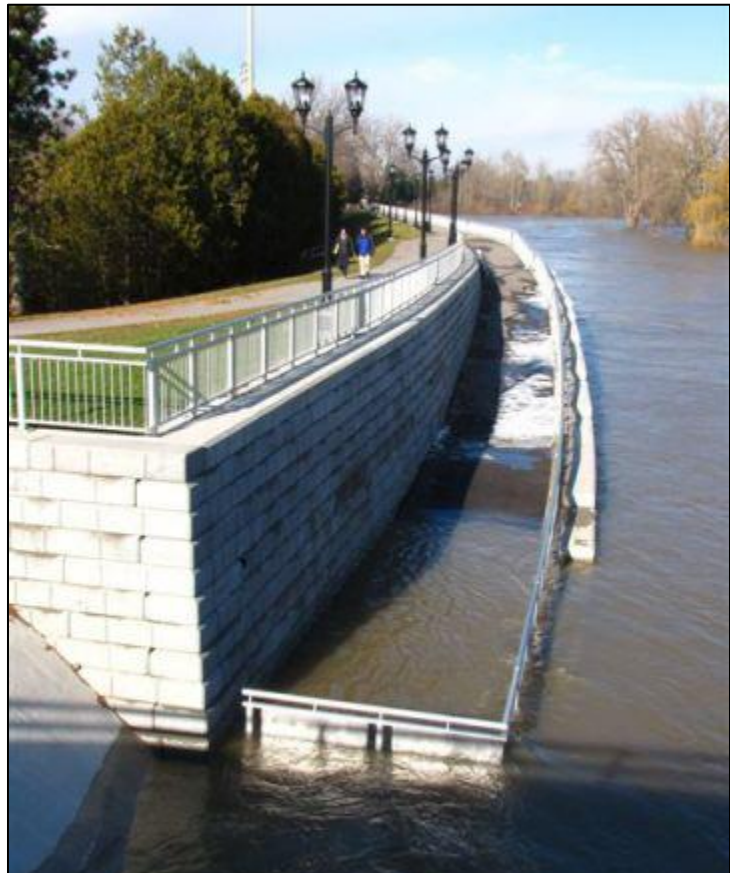
This wall is part of the Thames river levee system.
