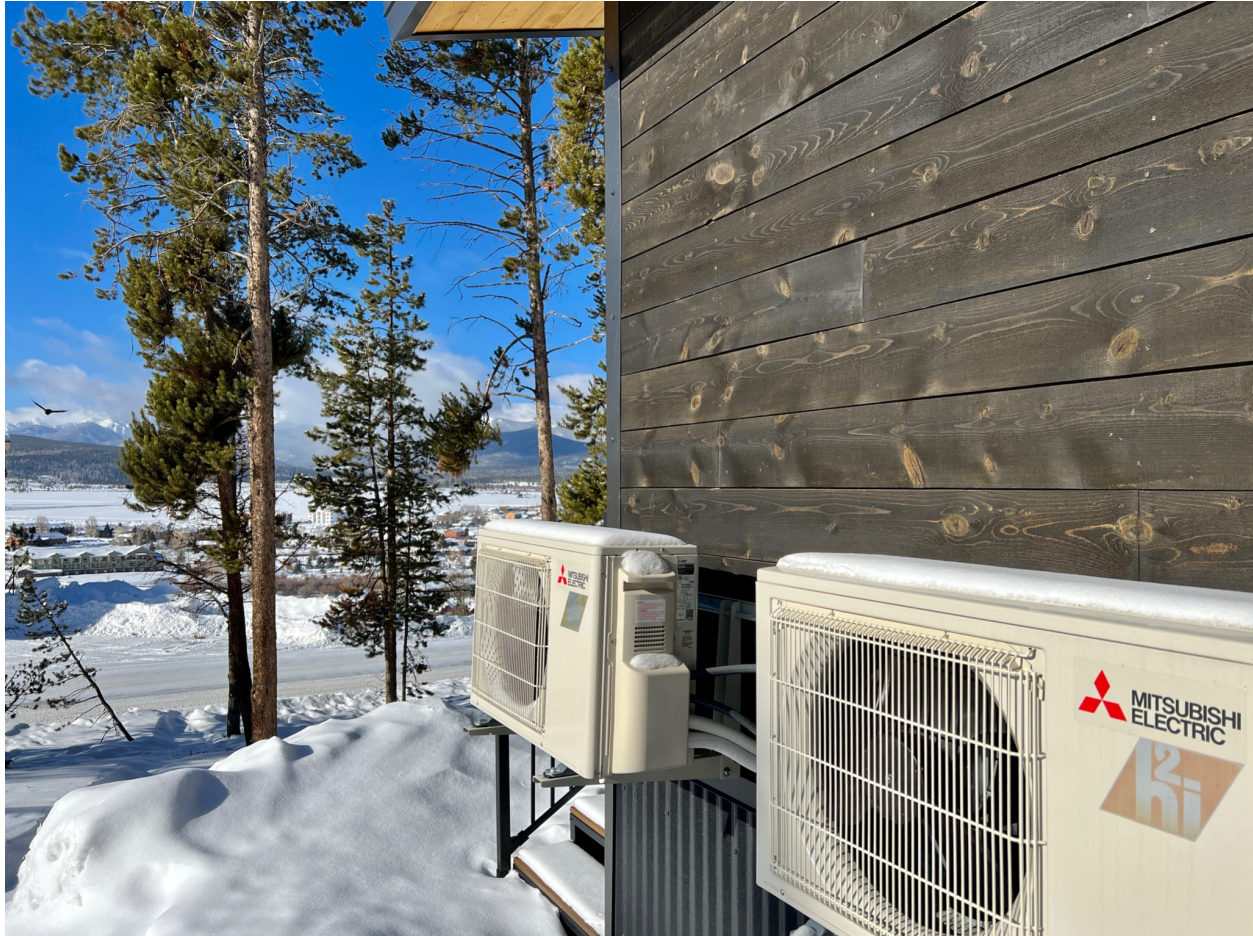
Picture 3. Cold-climate heat pumps heated the house during the first year without backup heat
