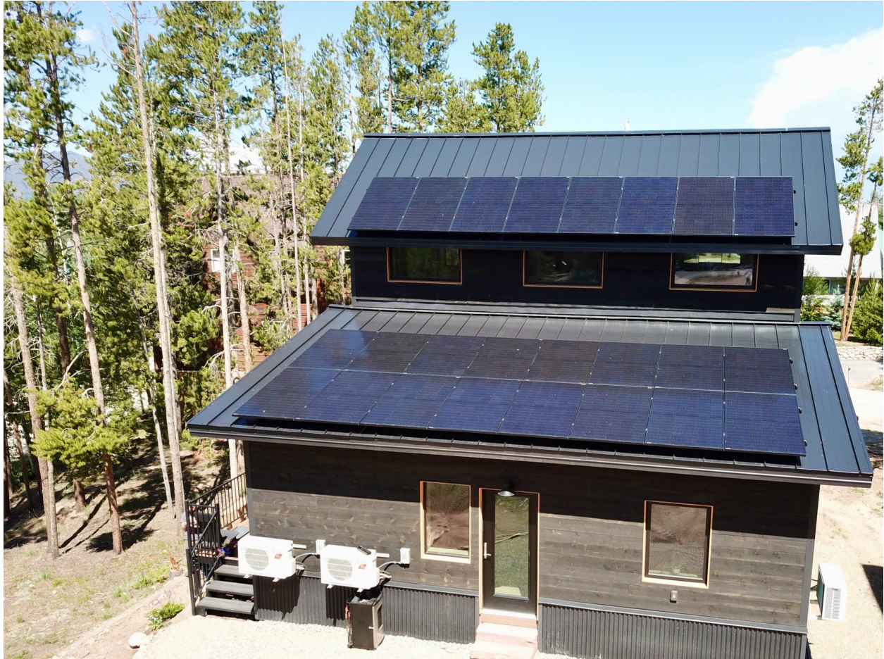
Picture 4. The 7.6 kW solar array generated 9.4 MWh during the first full year of operation
