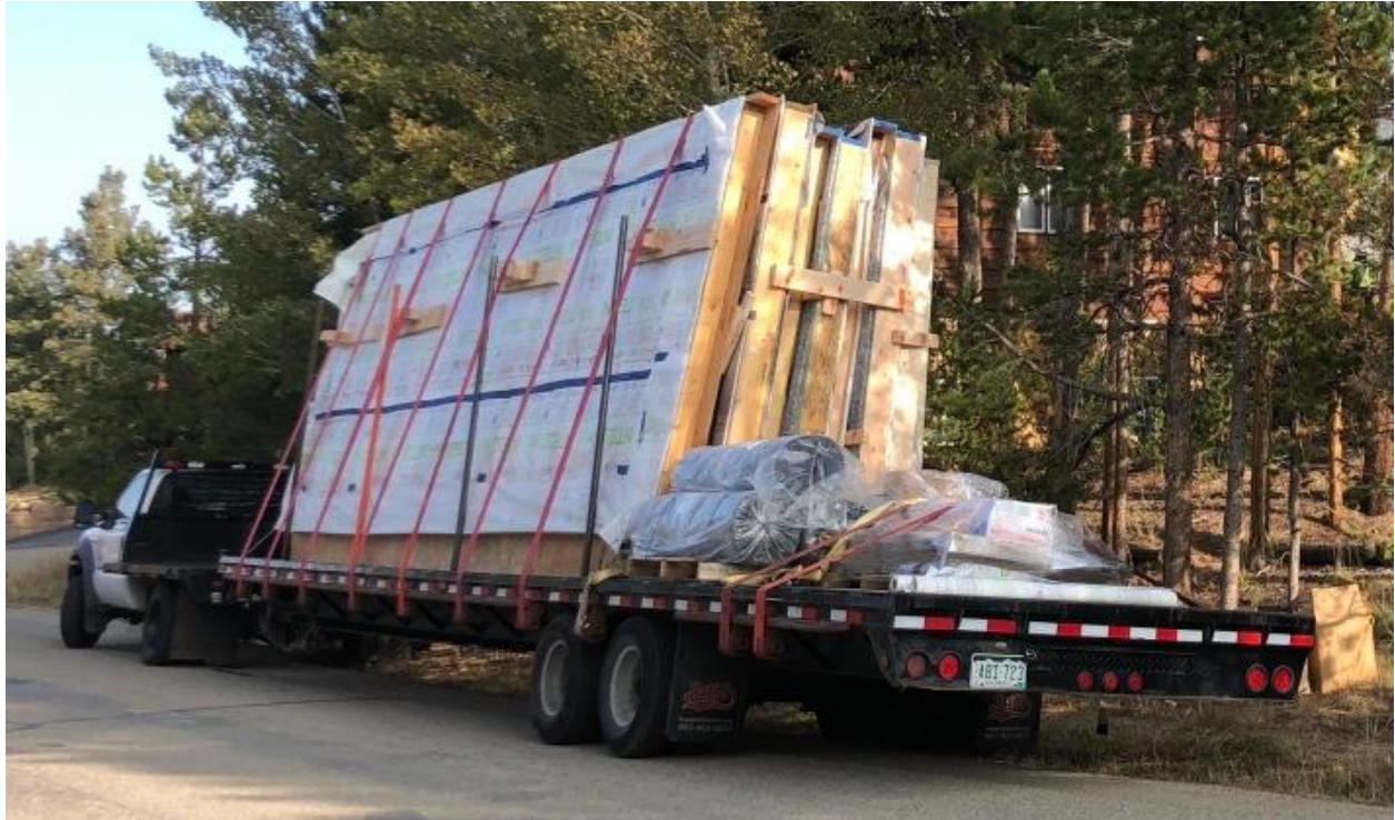
Picture 2. The SPARC House panels were pre-fabricated at Simple Homes in Denver and transported via truck in sections for modular assembly in Fraser
