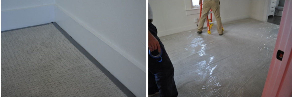
Figure 2: Duct tape used at the perimeter of carpeted rooms as a base for attaching the plastic covering (left). Plastic covering on carpeted floor (right).
