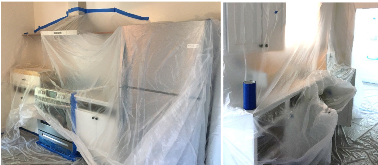
Figure 3: Kitchen appliances and cabinets covered for sealing. Photo on right shows cabinets opened to allow aerosol to seal plumbing penetrations and outlets below the sink.
