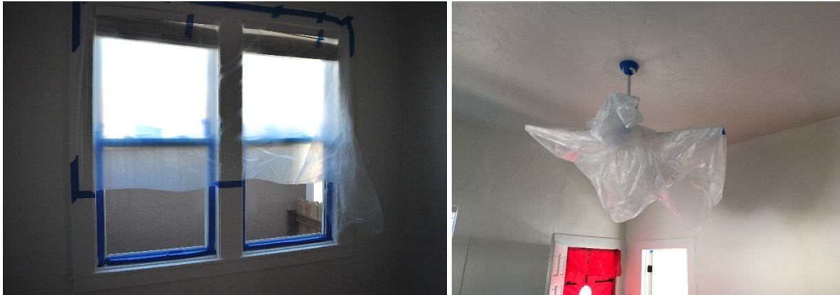
Figure 4: Windows prepped (left) and ceiling fan covered to protect from sealant deposition
