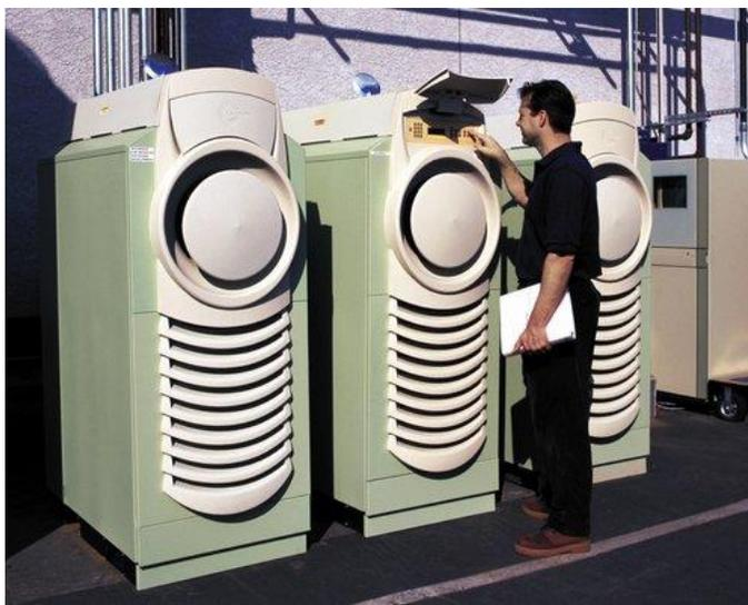
Figure 2. Set of three microturbines. Image courtesy of DOE/NREL. Credit: Capstone Turbine Corporation.
