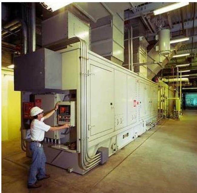
Figure 4. Gas turbine CHP system at Bristol-Myers Squibb in Wallingford, CT. Image courtesy of DOE/NREL. Credit: Bernard Blessinger.
