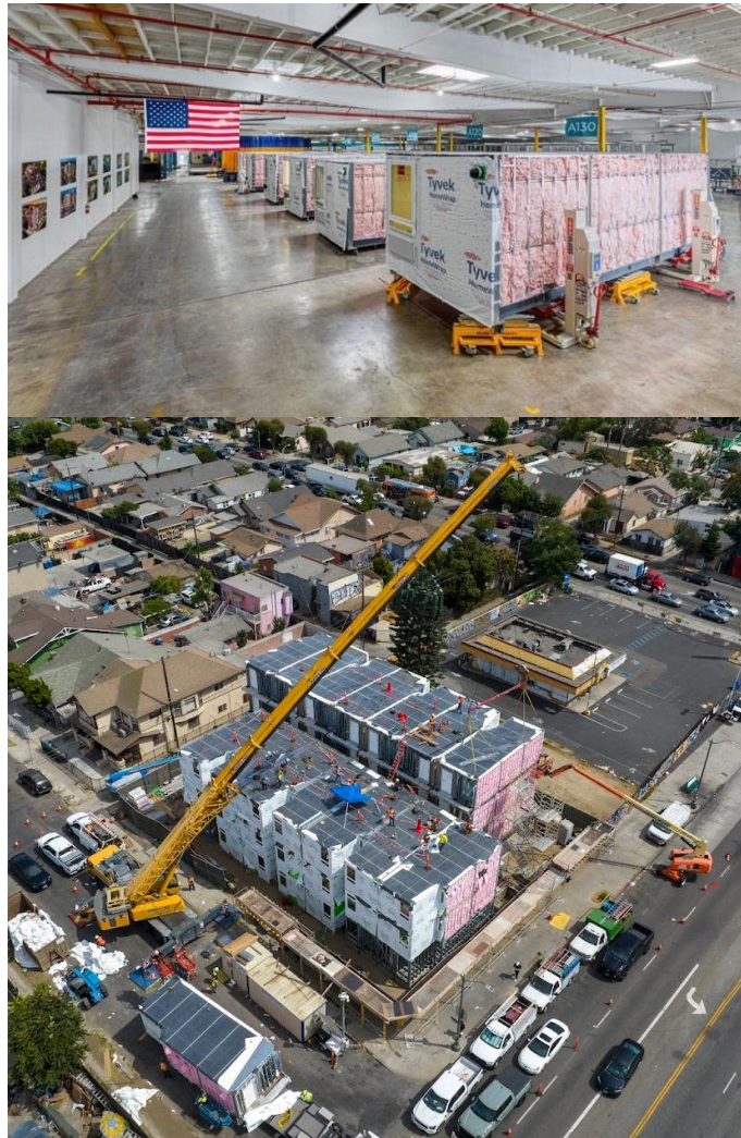
Figure 1. One-bedroom modular units ready for shipping (top) and during site assembly (bottom). These units are a successful example of modular industrialized construction. Credit: Model/Z
