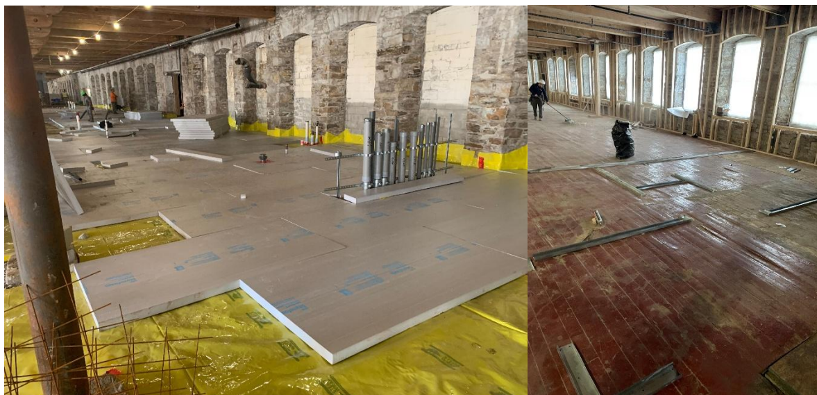
Figure 3 shows interior work and unit track layout during the renovation of Stone Mill.
