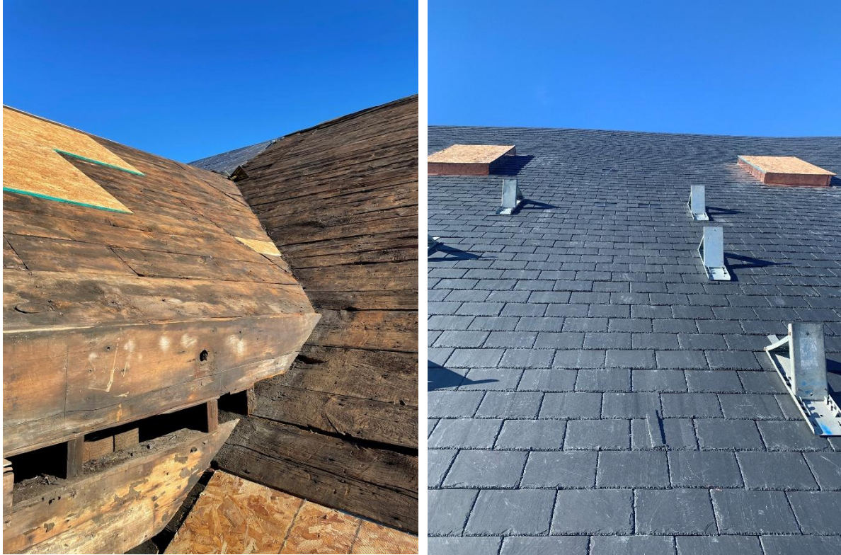
Figure 2 shows the baseline condition of the Stone Mill roof (left) and the new roof (right).
