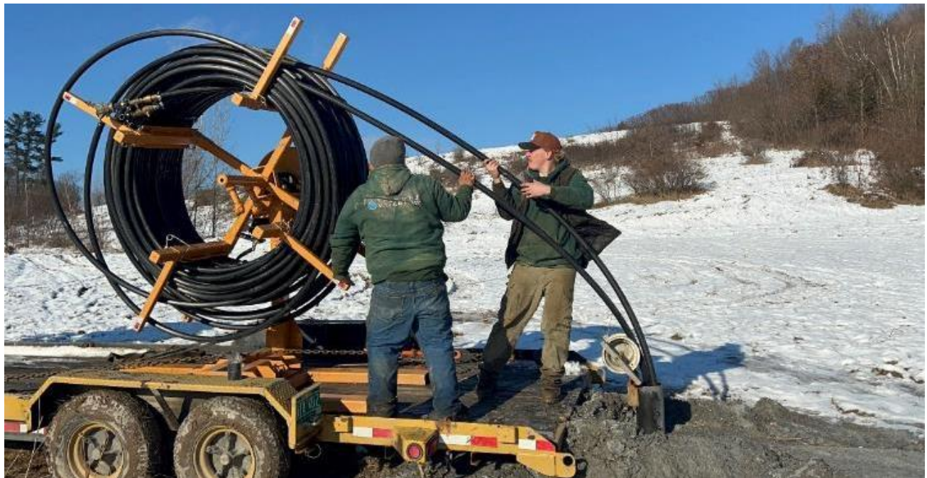
Figure 3. Polyethylene pipe being inserted in the borehole creating during construction of the borehole heat exchanger used for the thermal response test.
