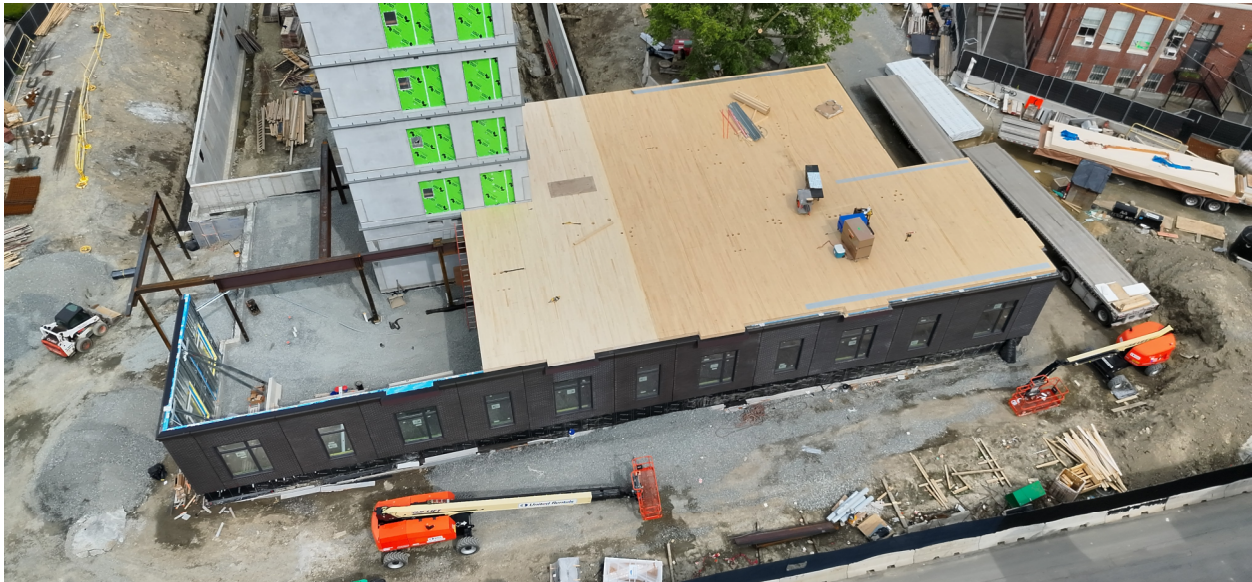
Figure 3. Construction photo of Building F, showing installation of the kit of parts: precast concrete cores, 64'-0" long 7-ply cross laminated timber floors, and fully clad load bearing wall panels.
