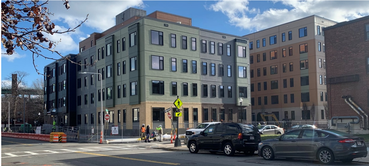
Figure 2. Completed view of the Phius-certified multifamily building M at the Bunker Hill Housing Redevelopment, Charlestown, Massachusetts.
