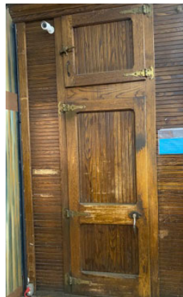
Figure 7. Original walk-in cooler with its historic ice box compartment above
