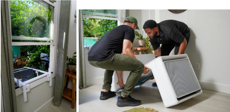
Figure 2. (left to right) Gradient's installation bracket in an open window; Two installers preparing to install the Gradient unit onto the bracket.
