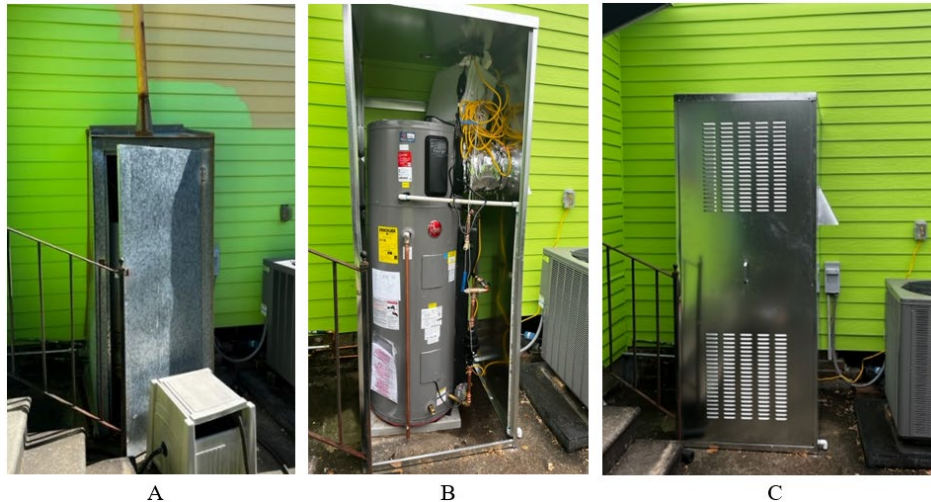
Figure 9. Replacement of a conventional water heater located in an outdoor enclosure (A) with a 120 V HPWH (B) in a new enclosure (C). Source: Pilet (2023).
