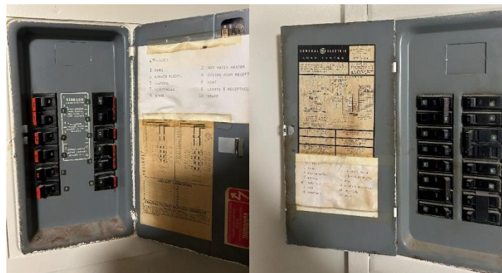
Figure 1. (Left) Federal Pacific Stab-Lok 12-space, and (Right) General Electric 16-space breaker panel.
