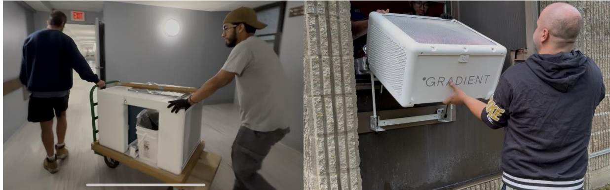
Figure 3. (Left) towing unit with cart to tenant unit (Right) positioning equipment in window.
