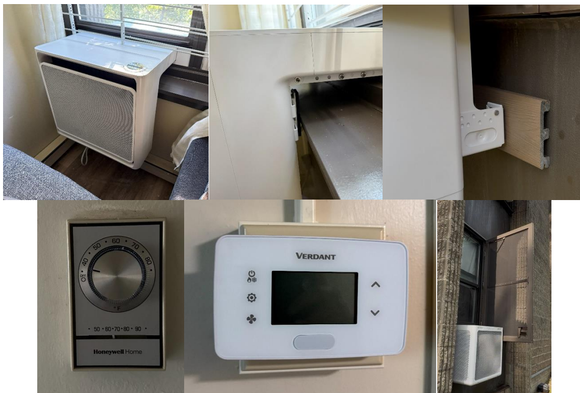
Figure 4. (Top-left) Final product in assembled in window, (Top-middle) product clearance with transition and interior windowsill, (Top-right) light-furnishing with PVC trim on exterior bracket leg, (Bottom-Left) old line-voltage thermostat, (Bottom-middle) newly installed Wi-Fi programmable thermostat, and (Bottom-Right) security screens pending removal.
