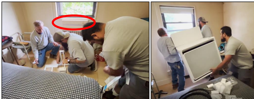
Figure 2. (Left) Bracket assembly also highlighting light carpentry work, and (Right) positioning equipment in window while maneuvering around furniture.
