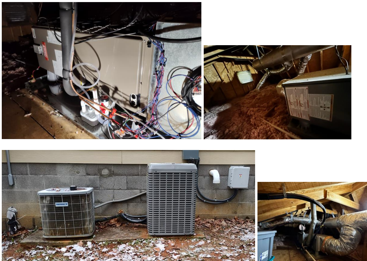
Figure 5. Details of field installation of the cascaded thermoelectric-integrated heat pump. (a) Top left: horizontal installation of indoor unit in the tight attic space. (b) Top right: undersized ductwork due to which return duct was replaced with a larger size. (c) Bottom left: Original AC for 1st floor, New heat pump outdoor unit for 2nd floor, and M&V Box installation. (d) Bottom right: Capped gas line and capped combustion vents in the attic.
