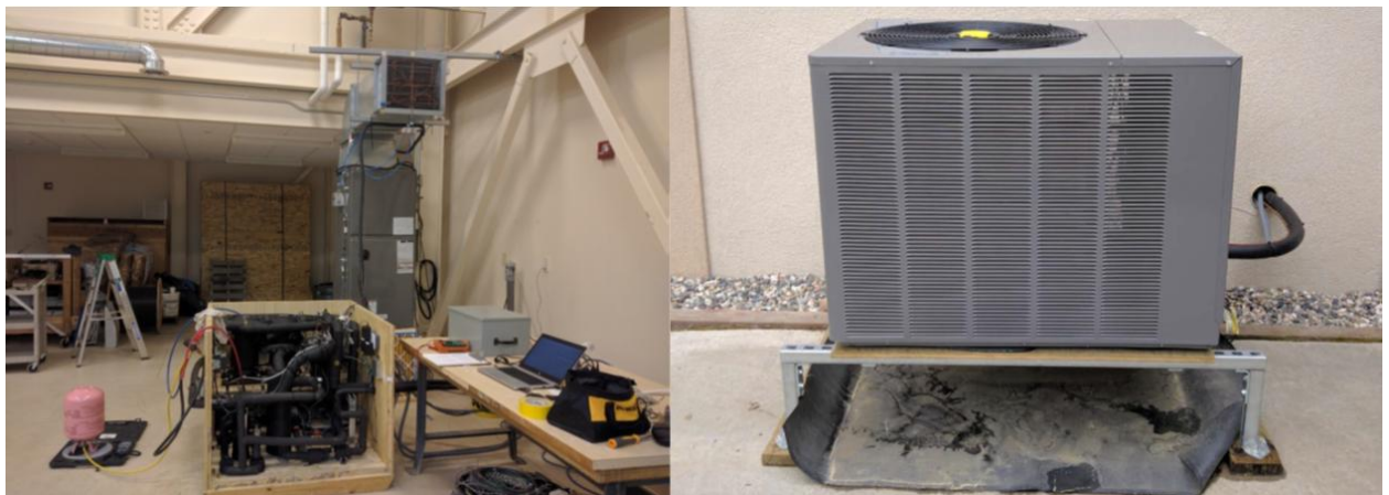
Figure 2. Field study of the CCHP using tandem compressors with vapor injection
