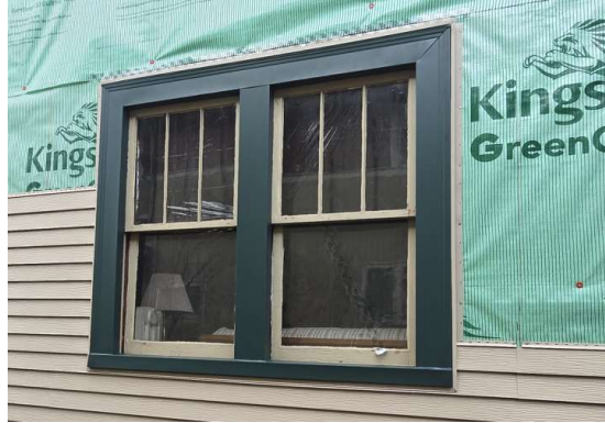
Figure 4. Window treatment where the edge of the CEI layer butts to a new lumber jamb extension that is wrapped in custom bent metal coil stock to provide a finished look. Source: PNNL, 2023.
