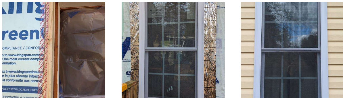
Figure 2. Window install where existing window is removed and lumber buck is placed to accept replacement window to meet new wall thickness. Source: PNNL, 2023.
