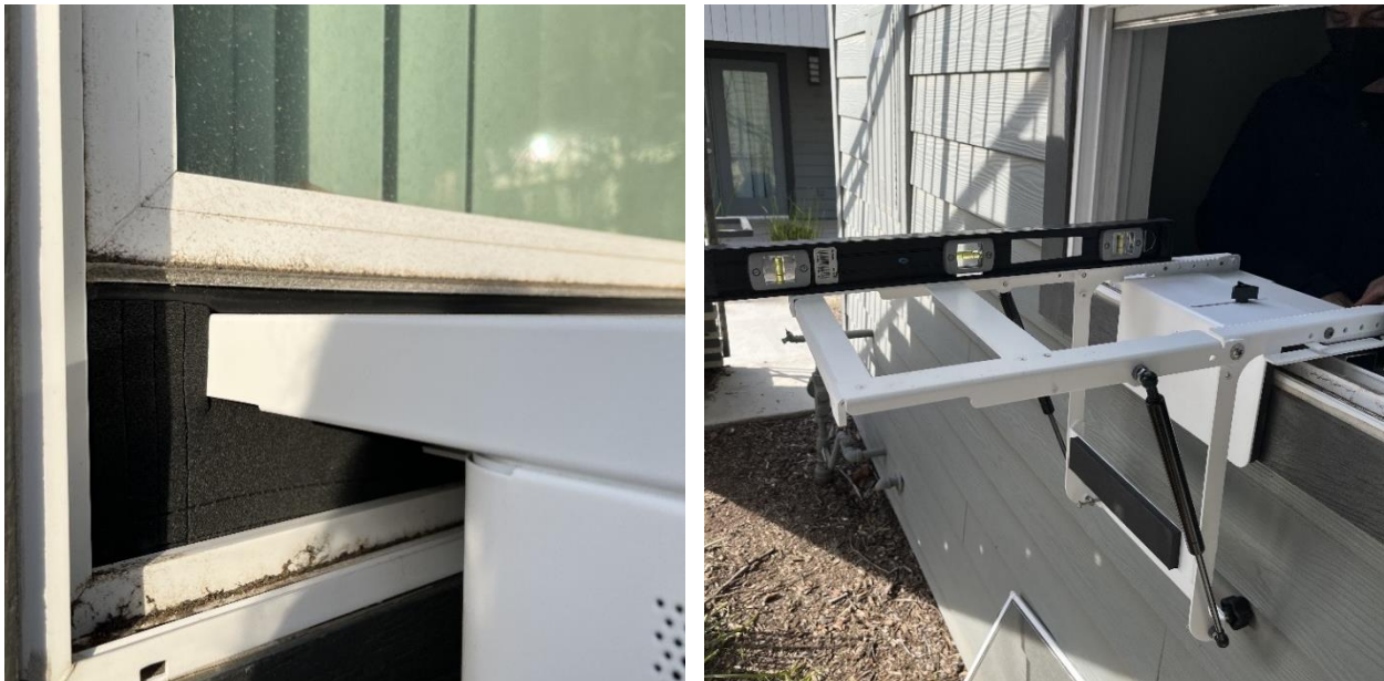
Figure 2: High density foam seal (left) and installation bracket (right).
