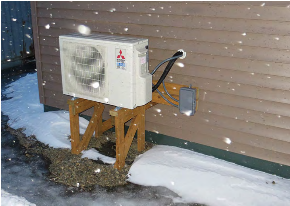
Figure 4. Outdoor unit of a ductless ccASHP in Dillingham, Alaska.
