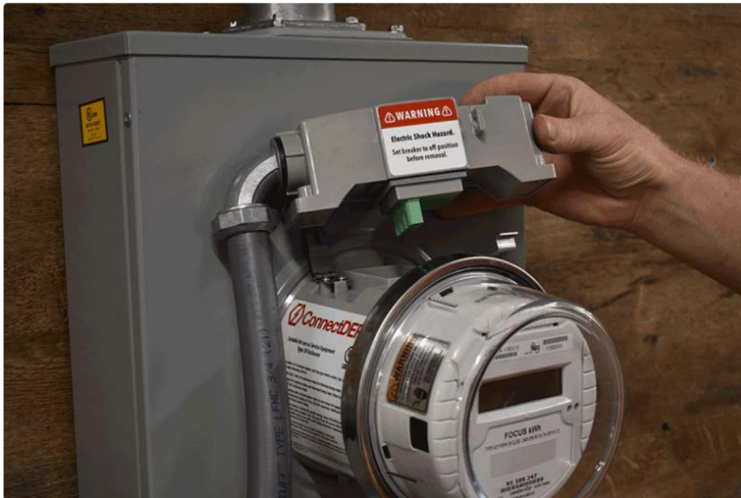
Figure 15. Meter collar that attaches to a home’s electrical meter. Source: ConnectDER web page ( https://connectder.com/ ).
