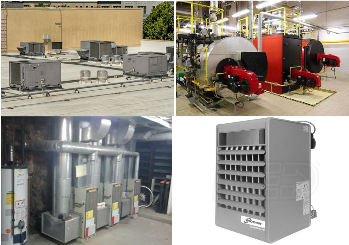
Figure 9. Illustration of different types of fossil fuel heating systems used in commercial buildings: gas-pack rooftop system (top left), boiler (top right), furnace (bottom left), and gas space heater (bottom right). Sources: Climate Control 2017; ASAP 2020; Dimare's Heating & Cooling Services 2020; eComfort 2020.
