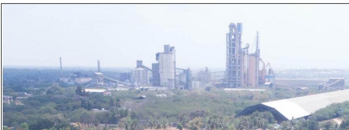
Figure 4: The Reddipalayam Plant in Tamil Nadu utilises AFR. Source: Ultratech Cement.
