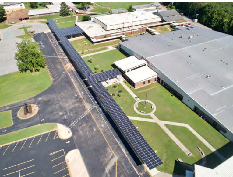
A solar canopy at a Batesville school district campus entrance. Source: Entegriety .
