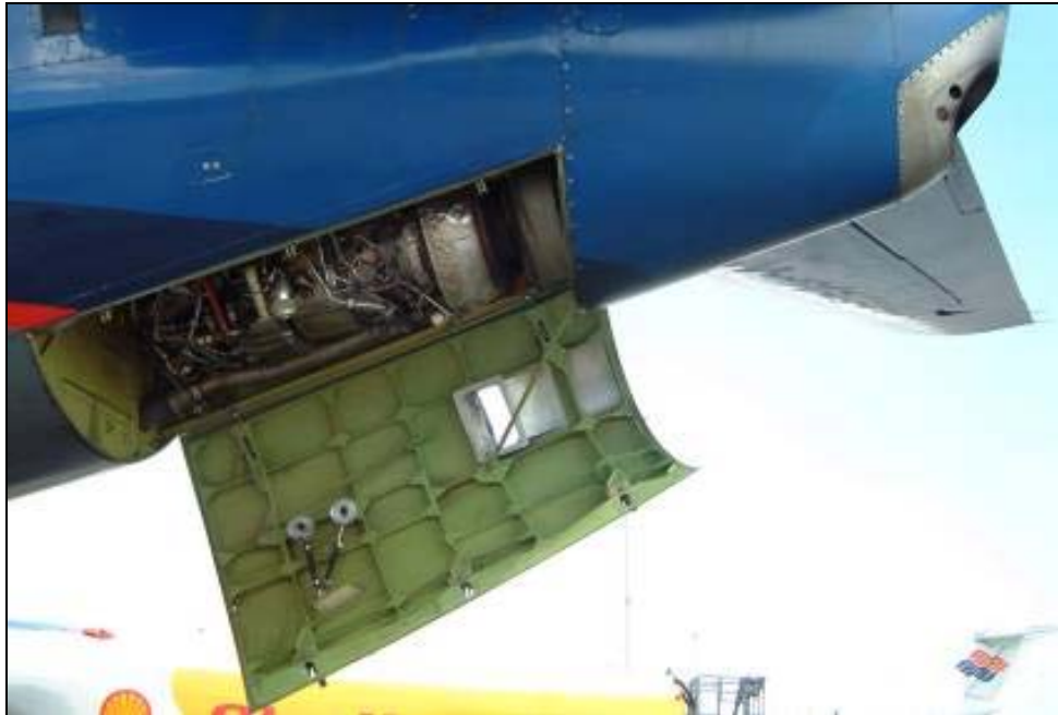
Figure 20: Auxiliary Power Unit
