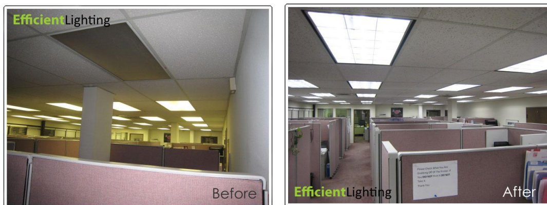
Figure C.4 Example of Improved Lighting Appearance with Energy Saving Lighting Retrofits (Efficient Lighting, 2008)
