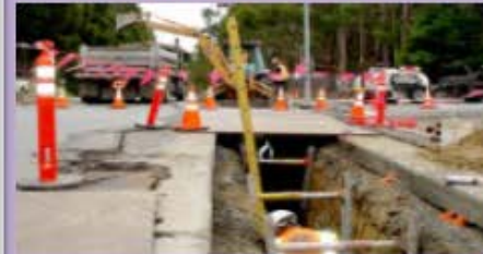
In-basin transmission system upgrades
