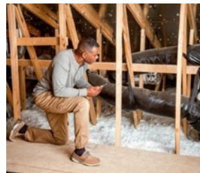
Attic & Wall Insulation
