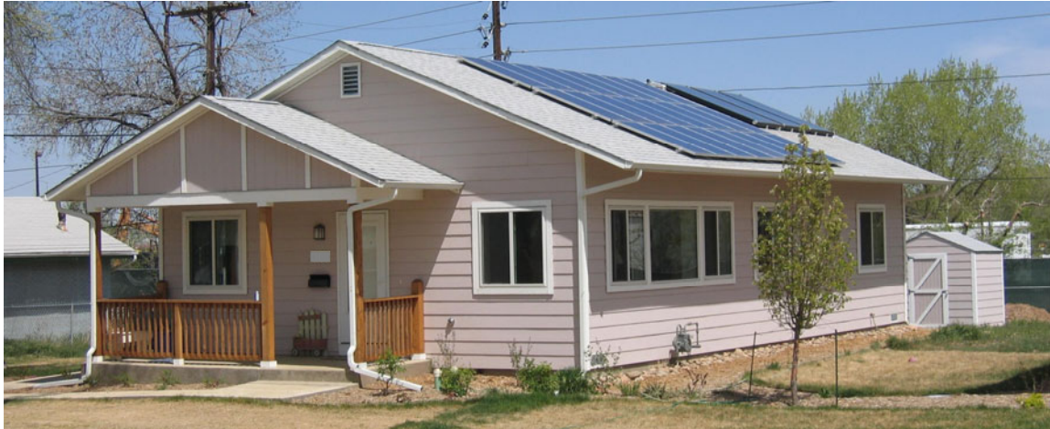
Figure 1. The Net-Zero Energy Habitat for Humanity House in Wheat Ridge, CO.
