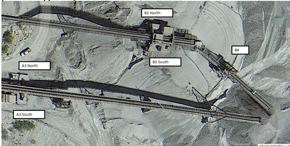
Figure 2. Image of overland conveyors.
