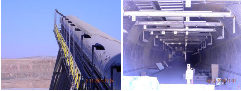
Figure 3. Left to right: external LEDs at crushing facility, internal LEDs at crushing reclaim tunnel.
