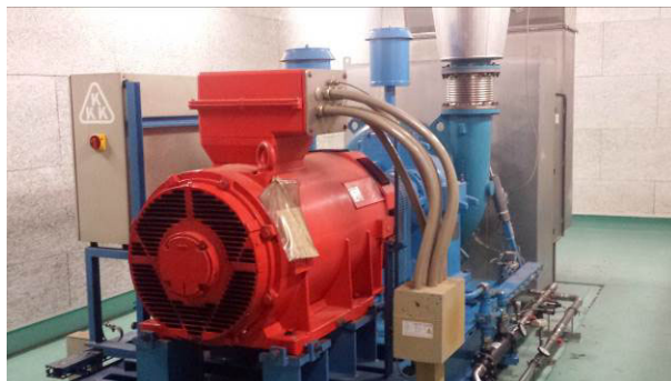
Figure 12. Motor system for turbo compressor.
