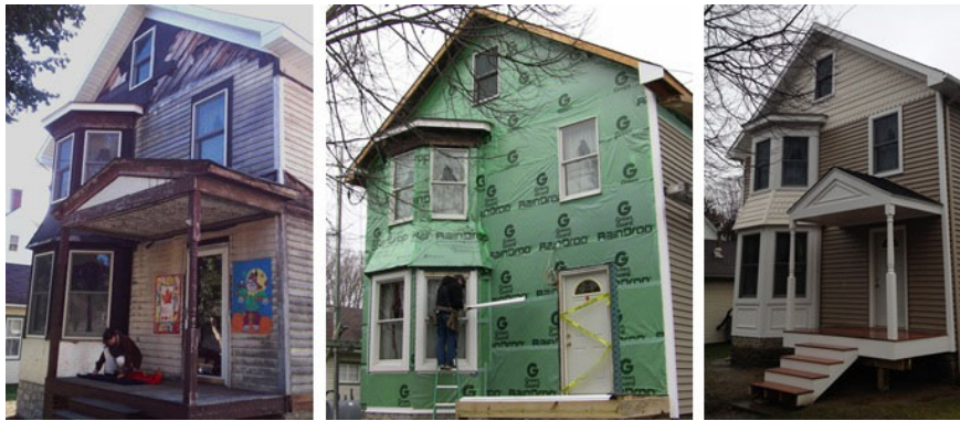
Figure 2. Example WRB Installation. Photos, Liaukus, C.
