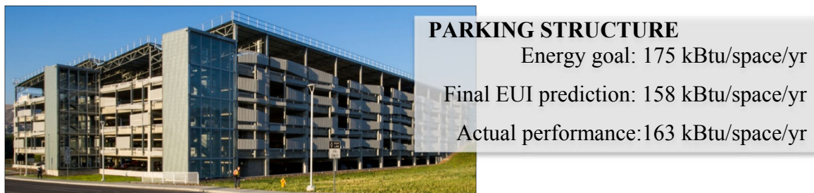
Figure 6. Northeast perspective image of the parking structure. Source: images.nrel.gov # 22471.
