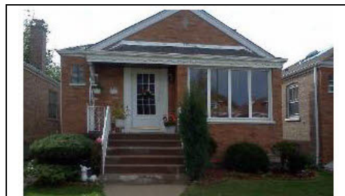
Figure 2. Photo of typical masonry home built between 1942-1978 less than 2 stories in Cook County, IL (group 4).
