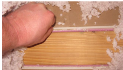
Figure 2. Attic view of sill sealer. Source: Bruce Manclark.
