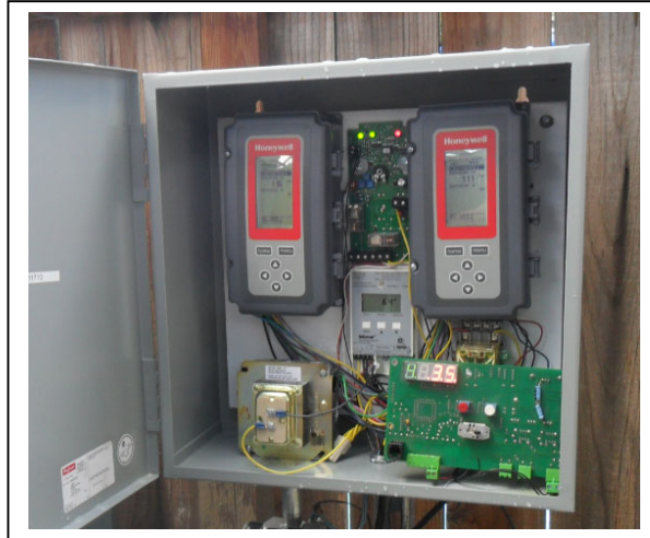
Figure 3. Photograph Of Controller As Deployed
