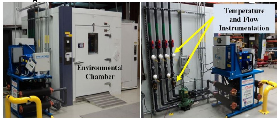
Figure 2. Installation of HRC with Environmental Chambers
