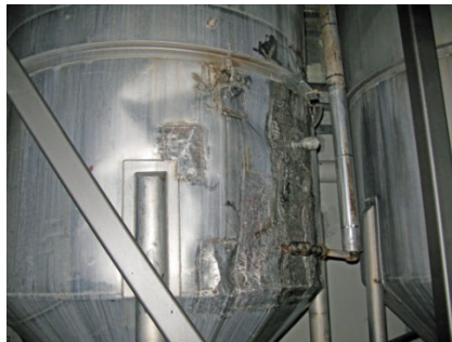
Figure 4: Damaged and Patched Sparge Tank
