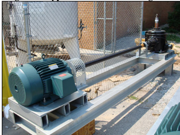
Figure 2. Typical Fan Drive Arrangement
