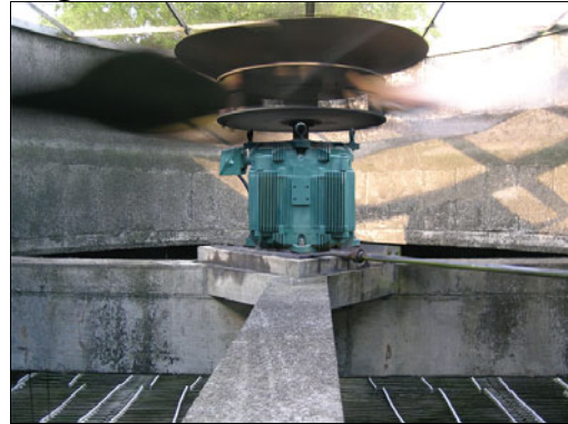
Figure 7. PM Motor Installed
