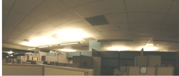
Figure 8. View of the Ceiling with Nearby Luminaires Turned Off
