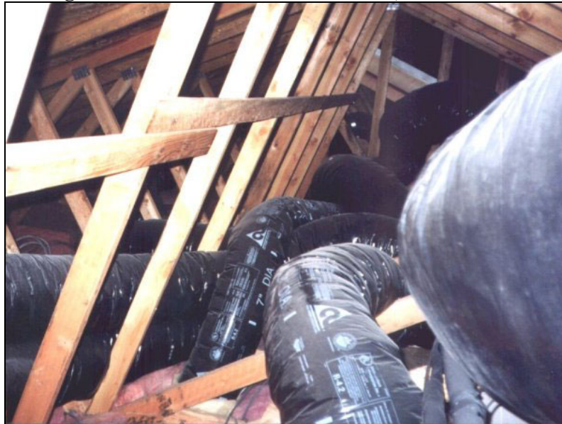
Figure 1. Ducts in an Unconditioned, Vented Attic
