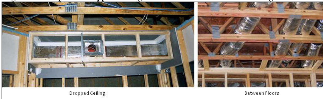
Figure 3. Examples of Dropped Ceiling and Between Floor Locations during Construction
