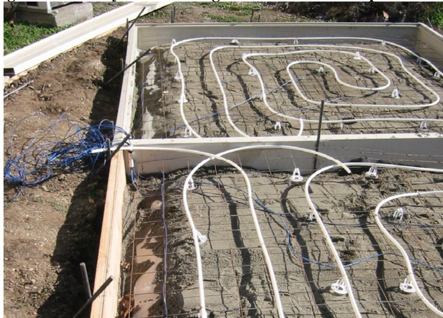
Figure 5. PEX Hydronic Tubing and Slab Thermocouple Installation
