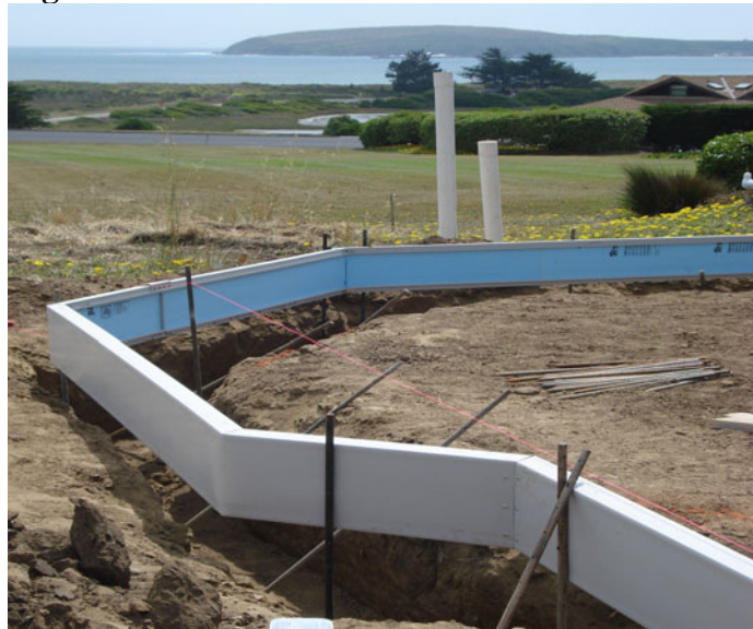
Figure 3. Insulated Form Board Field Installation
