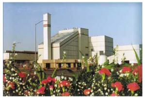
the facility processed 269,000 of the 356,000 tons of MSW not recovered for recycling or composting and therefore headed for landfills. The plant has an electric generating capacity of 26,000 kilowatts; the equivalent of supplying the electrical needs of 16,000 Washington homes. In 2007, the facility generated over 171,000 MWh of electricity.
