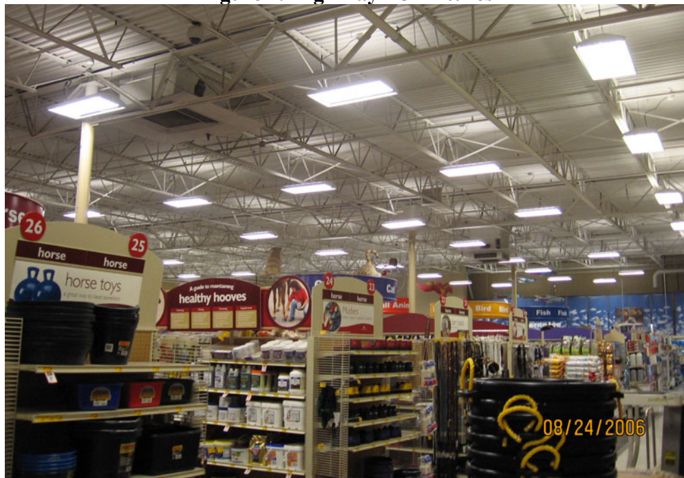
Figure 1. High Bay T8 Fixtures
