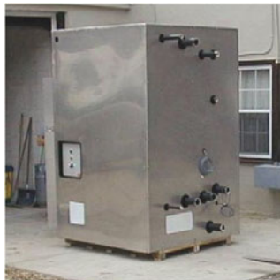
A 100 Ton chiller – 3.2 MMBTU/hr water heater unit.
