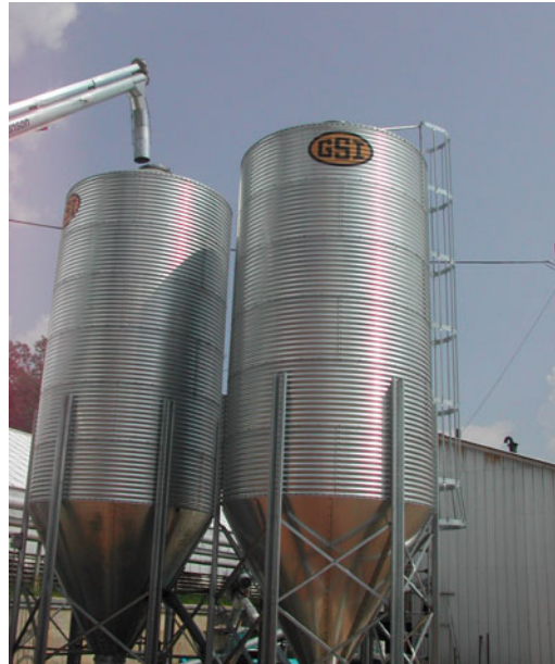
Figure 5. Bio-Mass Storage Tanks
